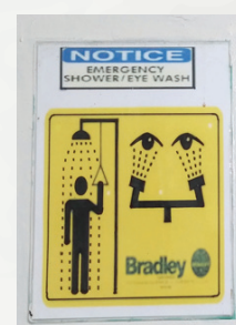
← The emergency shower
